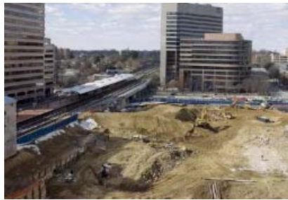
Christopher Anderson/The Gazette A view from the top of a nearby office building of the construction underway at the Silver Spring Transit Center at Colesville Road and Wayne Avenue in Silver Spring. Underground rock blasting has been underway for the past few weeks, to be followed by the first glimpses of the foundation and structure for the center. Expected opening date is June 2011.
